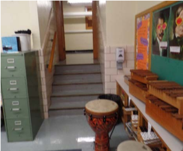
MERCER – INACCESSIBLE MUSIC ROOM
