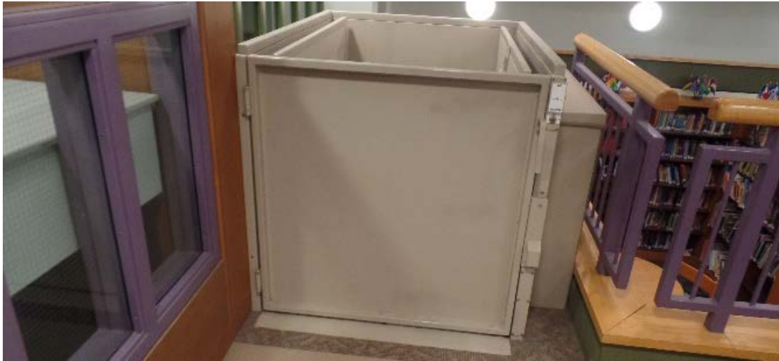
WOODBURY – LIBRARY LIFT
